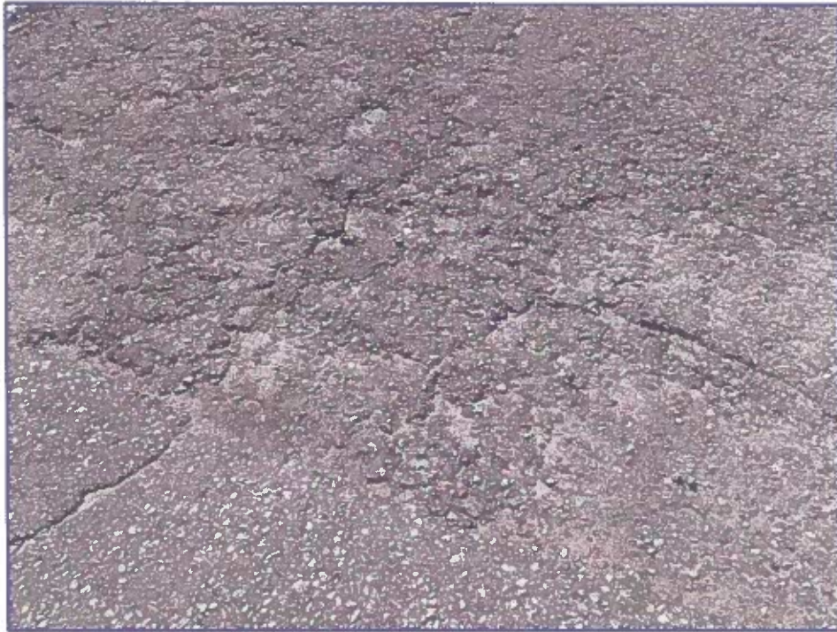
Photograph 21: Severely deteriorated asphalt at north side of site
