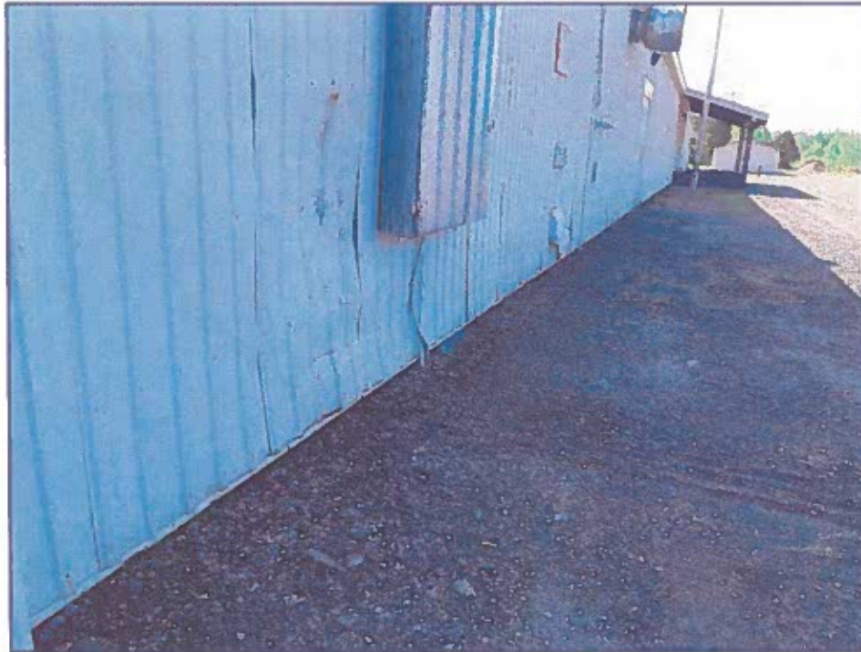
Photograph 13: Damaged steel siding throughout
