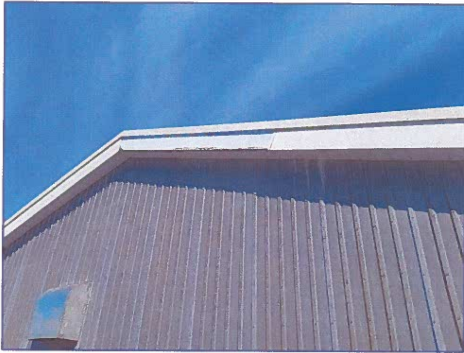
Photograph 19: Missing section of steel fascia on south face of roof
