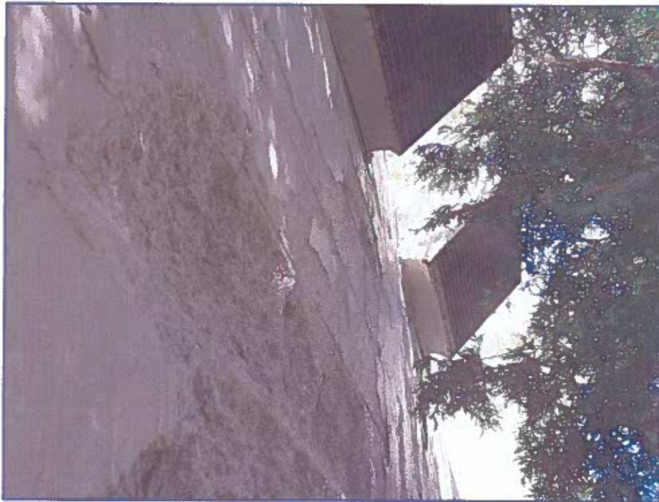
Photograph 20: deterioration of exterior block wall on east side of building as a result of moisture from vents above
