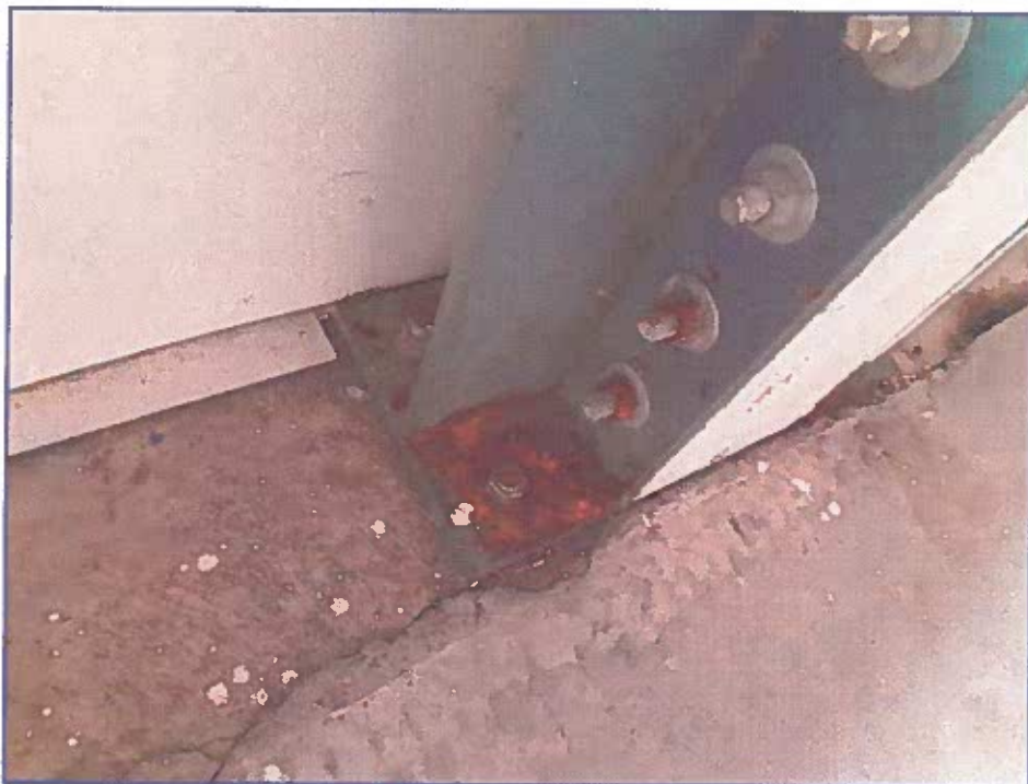
Photograph 12: Noted steel base plates which were reported to be installed in or around 2008 at the bottom of the wood columns starting to corrode, no section loss noted
