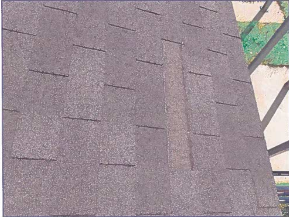
Photograph 17: Missing shingle on roof above Zamboni room
