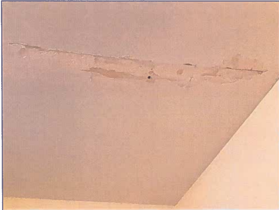
Photograph 5: Moisture damage in ceiling in women's washroom, previous leak reported to be repaired
