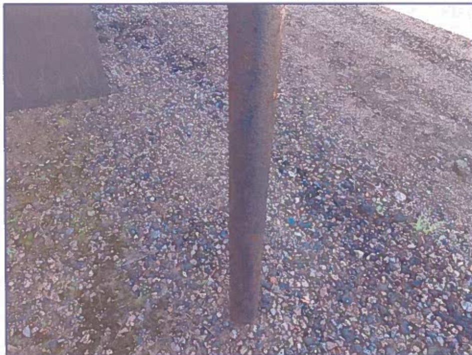
Photograph 14: Minor corrosion of steel posts supporting west roof overhang
