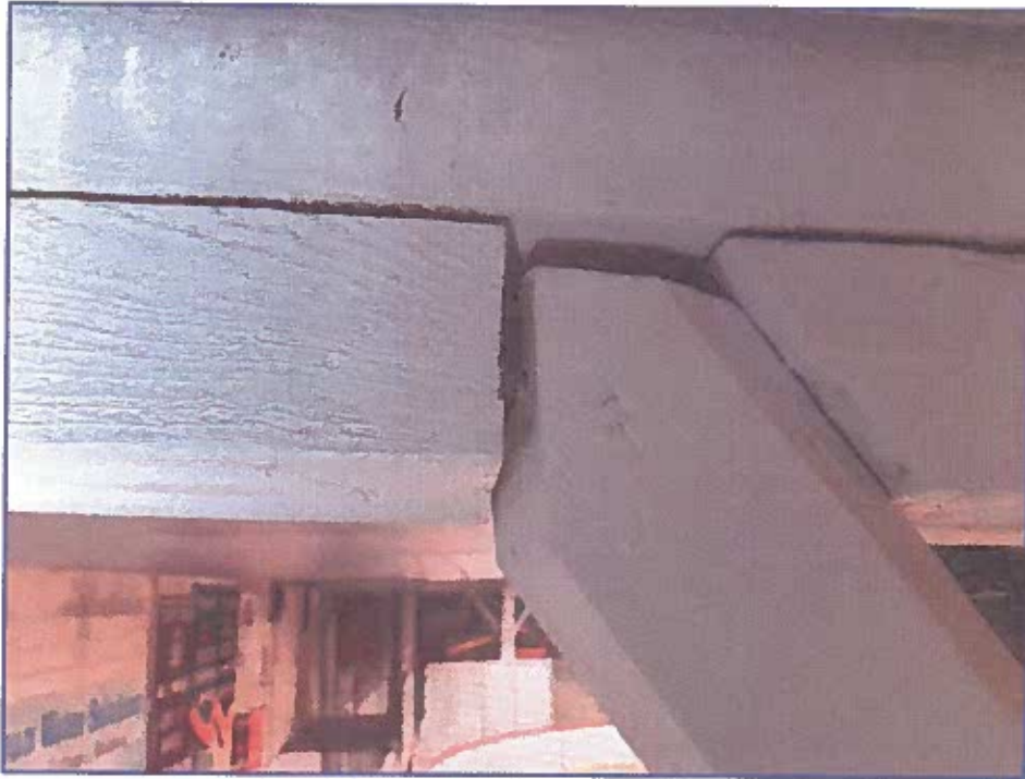
Photograph 11: Knee brace to roof beam connection is separating at southwest corner of structure
