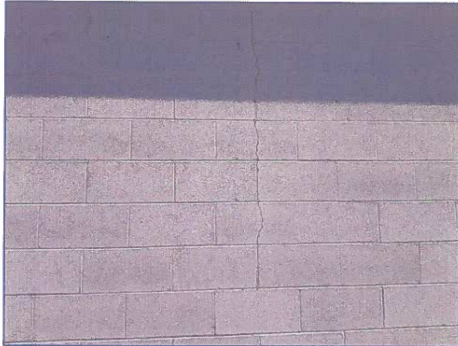
Photograph 16: Narrow vertical crack in south concrete block wall
