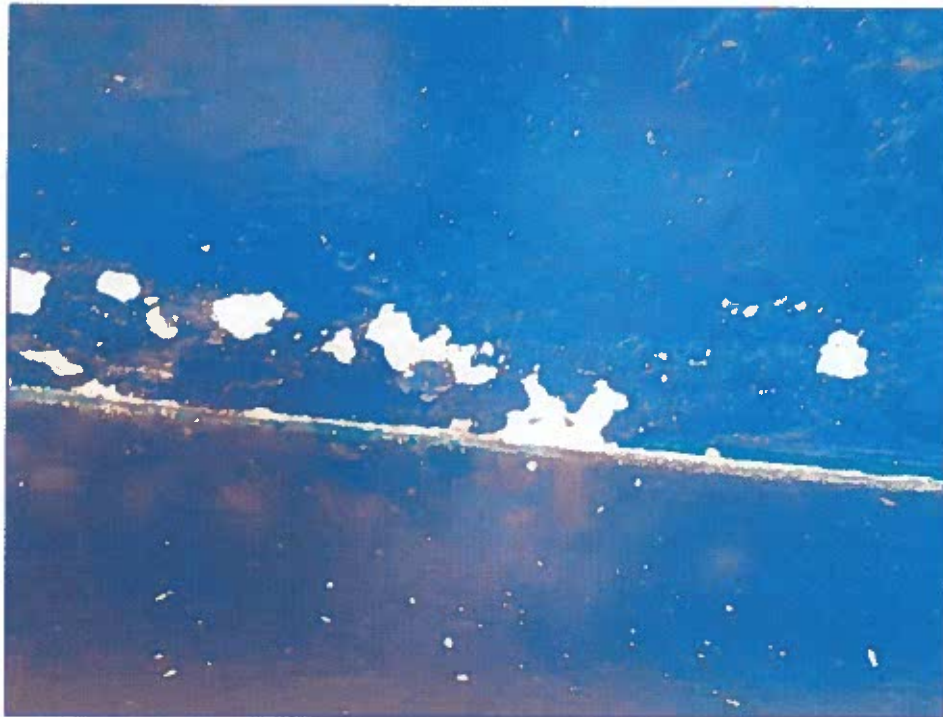
Photograph 8: Damaged parging and flaking of paint in dressing rooms
