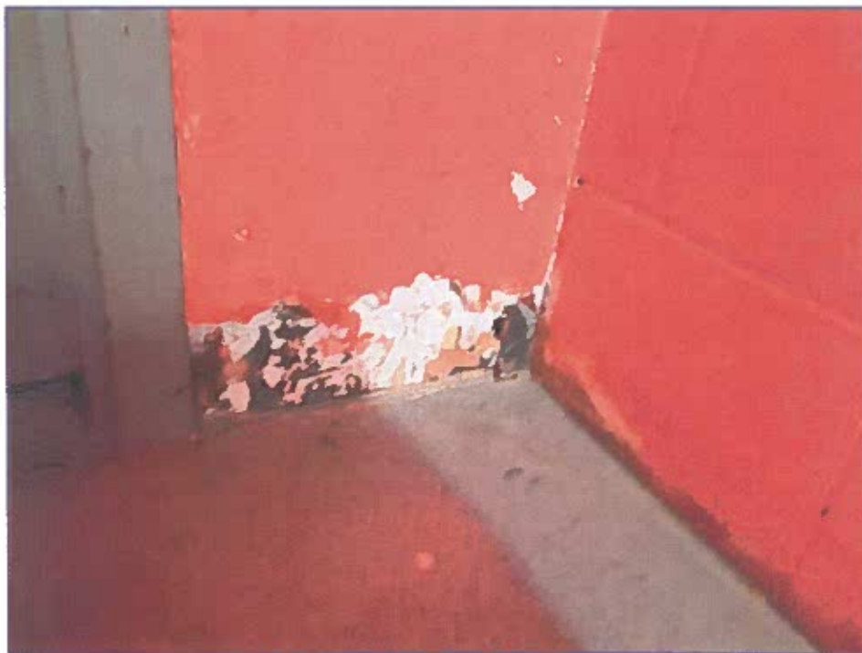
Photograph 6: Damaged drywall in hallway leading to dressing rooms
