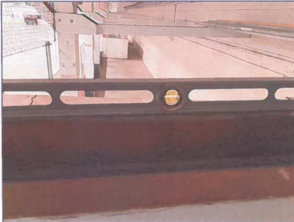
Photograph 10: Side bracing at southwest corner is sagging
