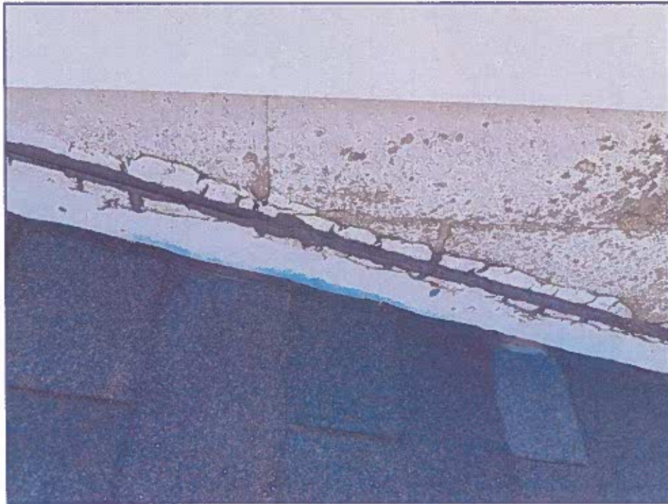
Photograph 18: Failing caulking throughout
